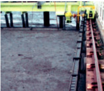
igus® lbt flizz® - Sewage works of the company Hydrobudowa S.A. in Poland. The power supply system of the scrapers in 8 clarifiers was equipped with igus® e-chain® and lbt flizz®. The complete system runs directly over the clarifier. Advantages: ● Low-maintenance system ● Longer service life ● Enclosed trough, protection against snow and ice ● Space-saving compared to conventional system ● Compact and safe ● Travel (S) = 42 m ● Assembled with igus® chainflex® cables
