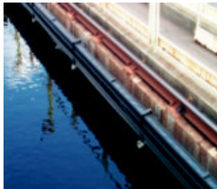
igus® lbt flizz® - Sewage works of the company Hydrobudowa S.A. in Poland. The power supply system of the scrapers in 8 clarifiers was equipped with igus® e-chain® and lbt flizz®. The complete system runs directly over the clarifier. Advantages: ● Low-maintenance system ● Longer service life ● Enclosed trough, protection against snow and ice ● Space-saving compared to conventional system ● Compact and safe ● Travel (S) = 42 m ● Assembled with igus® chainflex® cables
