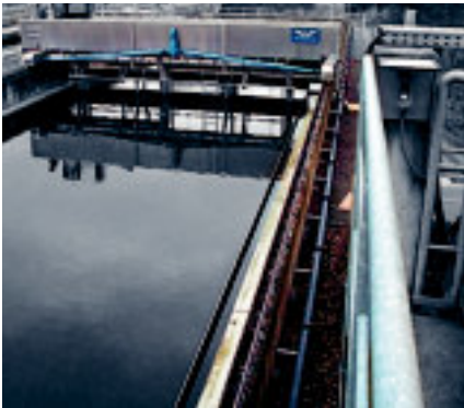
lbt flizz® in a longitudinal scraper travel (S) = 38 m
