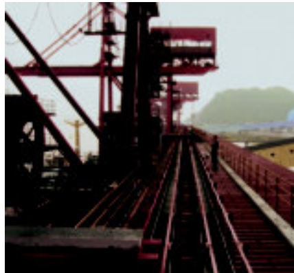
Series 4040R on a coal unloading system - Travel 190 m, Speed 0.5 m/s, Fill weight 8.05 kg/m
